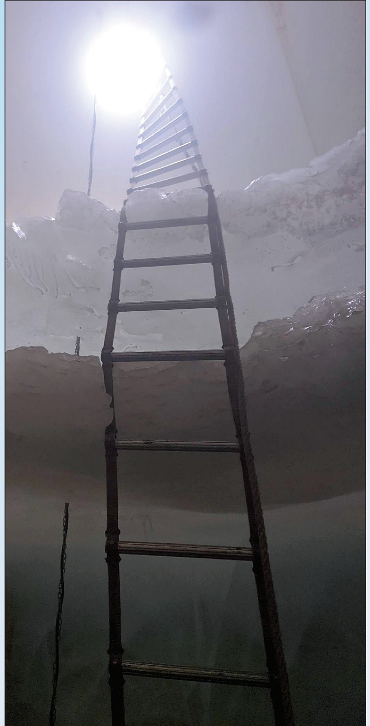
Tower complications due to cold temperatures.
